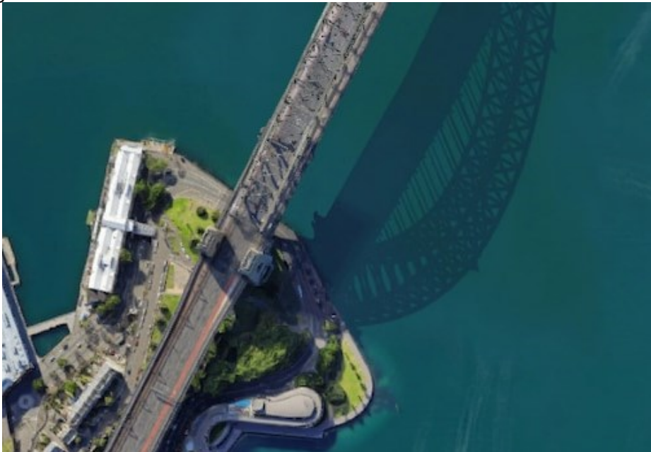
Figure 16 The shadow of the bridge tells us something about its structure
