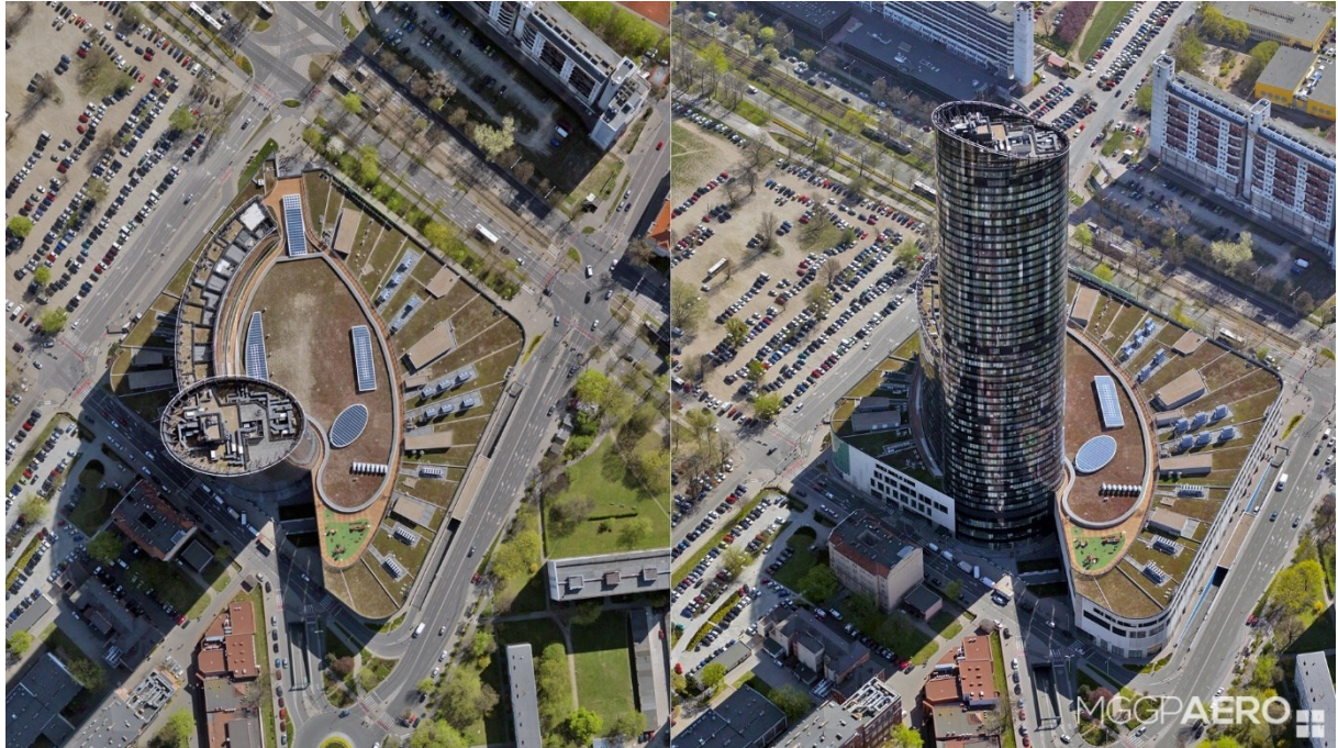
Figure 14 In the oblique images we can for example measure the building height or count the floors.
